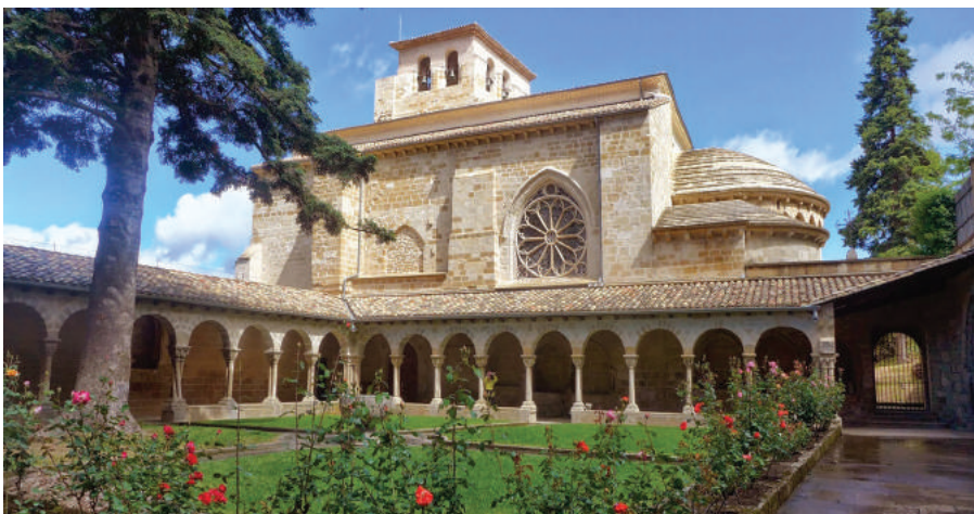
Church of San Pedro de la Rúa, Estella, photo by Amawalker
