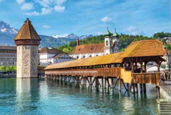
As the oldest wooden bridge in Switzerland, the beloved Chapel Bridge, built in 1333 and adorned with paintings of historic Lucerne.
